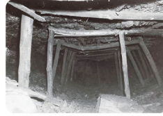
갱목이 부러진 미이케탄광 미카와갱 내부 1945 Inside the Mikawa Pit of Miike Coal Mine, where the timbers supporting the tunnel were broken off
